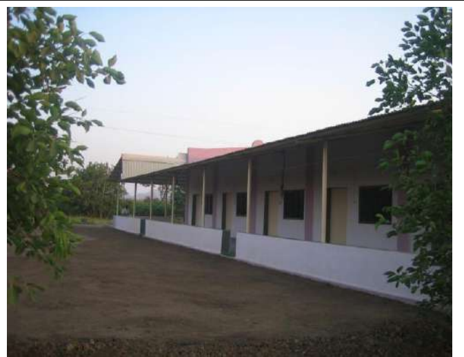
Residential Quarters for the Trainees
